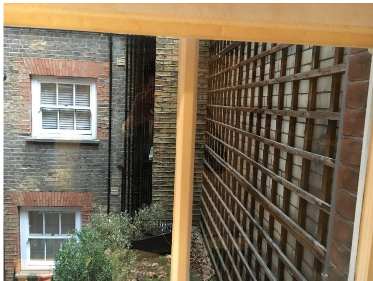
Rear Elevation Viewed From South at a Right Angle
